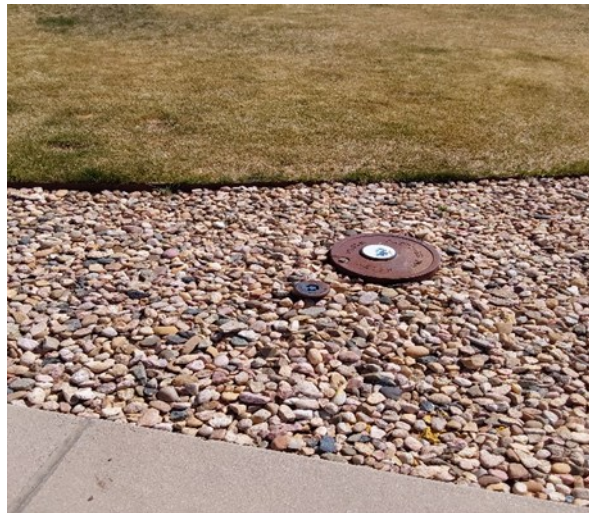
Accessible meter pit lid and curb stop.
