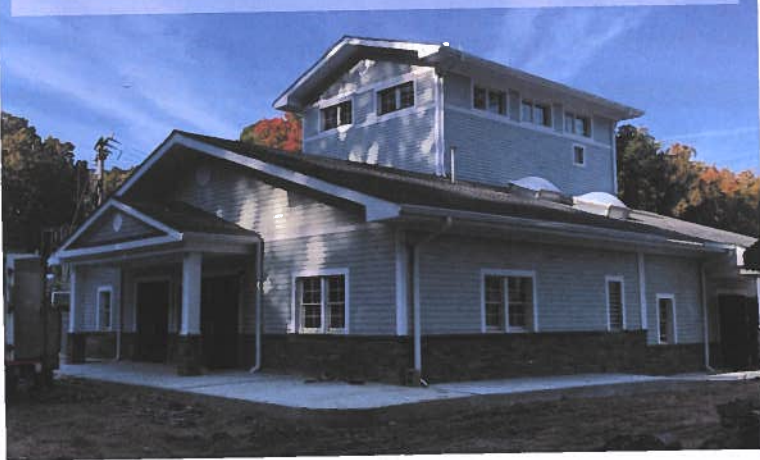
New Treatment Center at the JWD Water Tower is nearing completion
